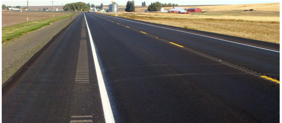
Shoulder rumble strips and center line rumble strips are installed on this roadway.
