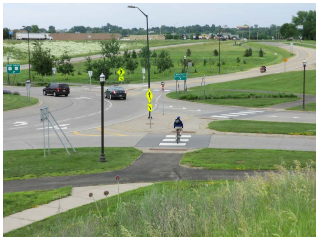
Example of a multi-lane roundabout.
