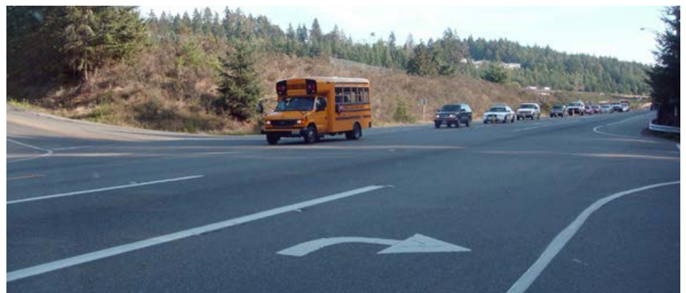
Example of a right-turn lane.
