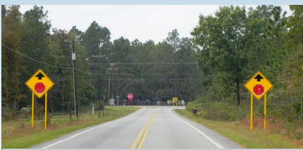
Example of countermeasures on the stop approach.
