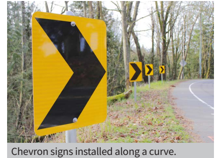
Chevron signs installed along a curve.
