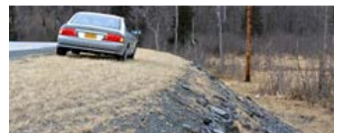
Shoulder is provided along roadway curve.
