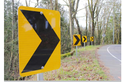
Chevron signs installed along a curve.
