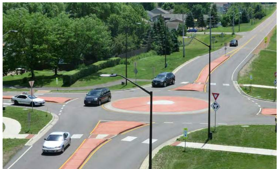
Example of a single-lane roundabout. Source: FHWA
