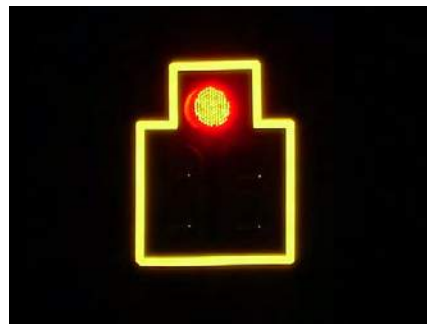
Retroreflective borders are highly visible during the night. Source: South Carolina DOT
