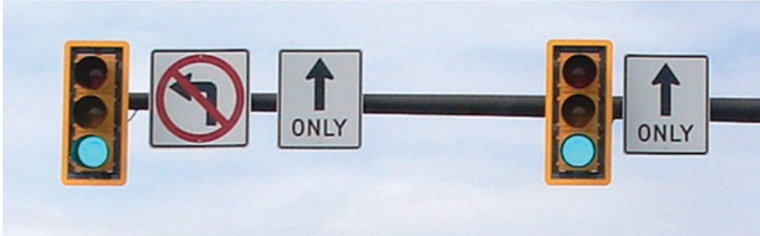
Figure 3: Signal retroreflective backplates [30].
