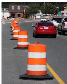
Courtesy of NJDOT, 2020.
